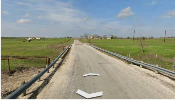
Figure 2 County Road 405 would be inundated by about 7.6 feet of floodwaters during a breach of Upper Brushy Creek FRS No. 29
