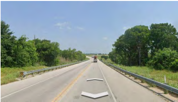
Figure 4 N State Highway 95 would be inundated by about 3.4 feet of floodwaters during a breach of Upper Brushy Creek FRS No. 29
