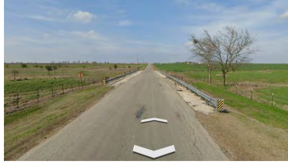
Figure 3 County Road 406 would be inundated by about 6.5 feet of floodwaters during a breach of Upper Brushy Creek FRS No. 29
