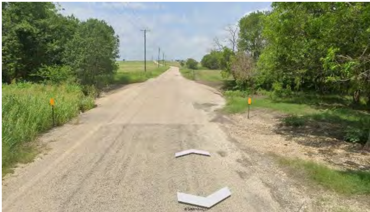
Figure 2 County Road 398 would be inundated by about 7.6 feet of floodwaters during a breach of Upper Brushy Creek FRS No. 25
