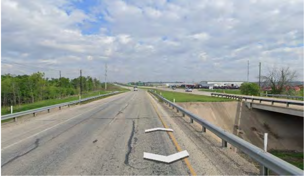
Figure 7 US Highway 79 would be inundated by about 2.7 feet of floodwaters during a breach of Upper Brushy Creek FRS No. 25
